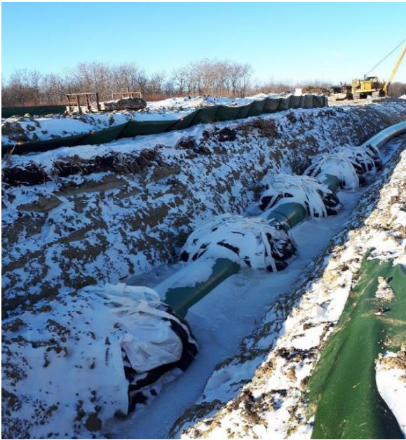
Eco bag weights placed on pipe in wetlands and coconut matting placed on top for wetland restoration
