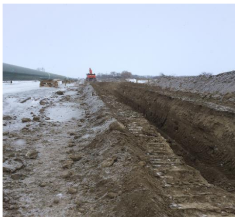
784 + 842 Excavating ditch lines
