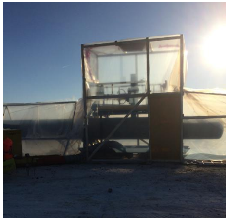
East side of the Pipestone Creek – Hoarding for test pipe string & removing test head.
