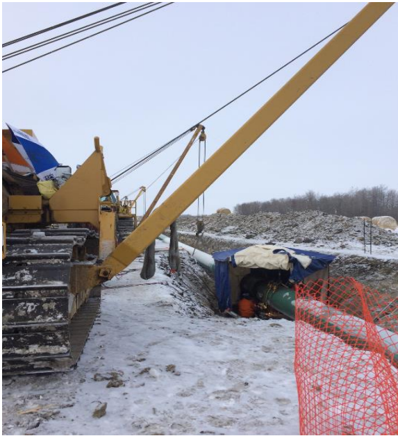
742 + 101 welder tying in pipe & 741 + 779 coating pipe
