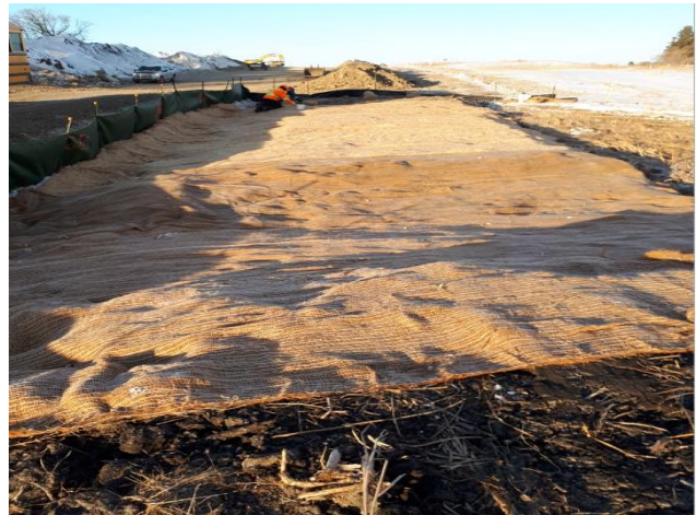
Eco bag weights placed on pipe in wetlands and coconut matting placed on top for wetland restoration
