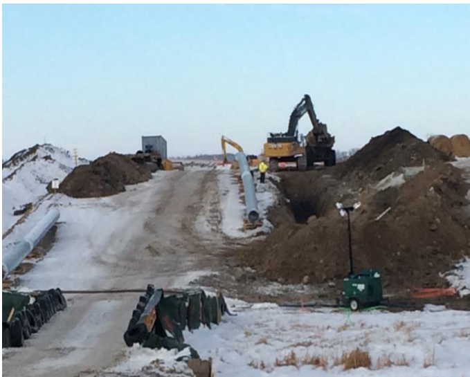
The Little Pipestone Creek Excavating ditch, Pumping water and sand pipe installation
